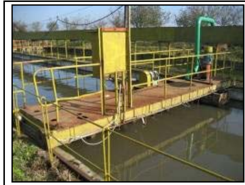
Figura 2.10-20: Decantor secundar
